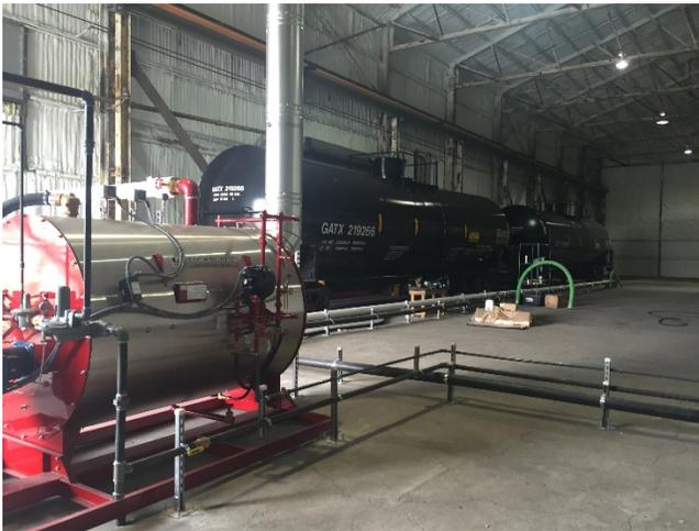
There are three main methods to heat a tank rail car for offloading or transloading: 1) hot water from an industrial water heater pumped through the heat lines of the tank car, 2) steam from a high-pressure boiler system, and 3) low-pressure steam from a steam generator. Hot water and high-pressure steam are used for very specific applications and facility layouts. Low-pressure steam from a steam generator is the most versatile when it comes to products to be unloaded and facility layouts.
