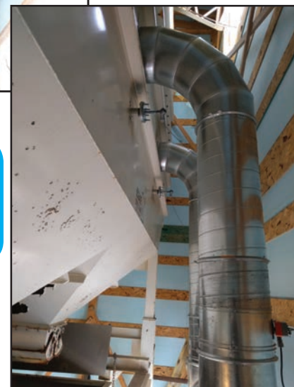
Heating Ducts Going into Aggregate Bins
