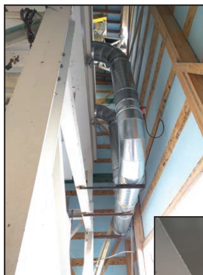
Heating Ducts Going into Aggregate Bins
