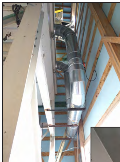
Heating Ducts Going into Aggregate Bins
