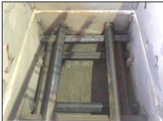
Heat Diffusers in Rock Bin & Sand Bin
