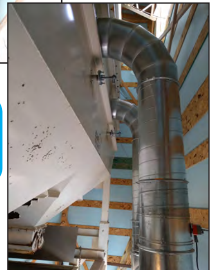
Heating Ducts Going into Aggregate Bins
